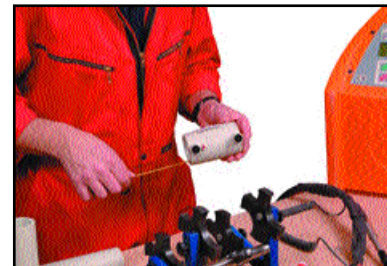
Measuring the fitting insertion depth
