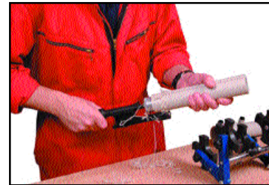
Peeling the pipe end prior to jointing
