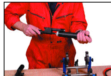
Peeling the pipe
