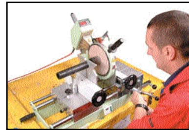
Heating the pipe and fitting
