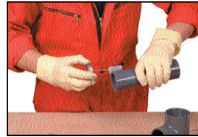
Applying the primer to the pipe
