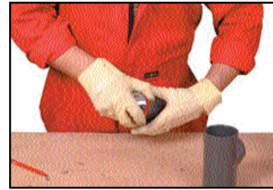
Chamfering the pipe
