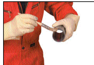
Brush applying cement to the pipe
