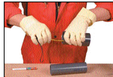
Measuring the insertion depth
