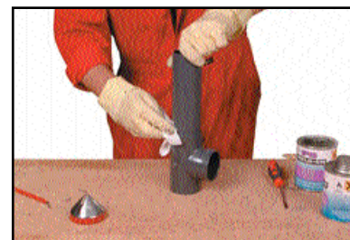
Wiping away excess cement
